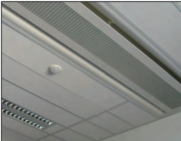
VFK 600 Chilled Beam Installation
